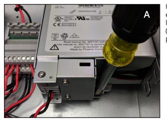
Use a flat-head screwdriver, or equivalent, to release the DIN-RAIL latch on the UPS battery. (Located in the upper right of the panel)
